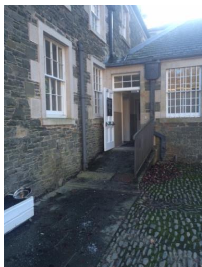
Access from Courtyard
