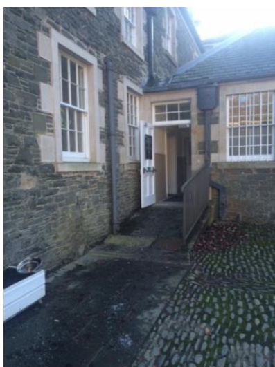
Access from Courtyard
